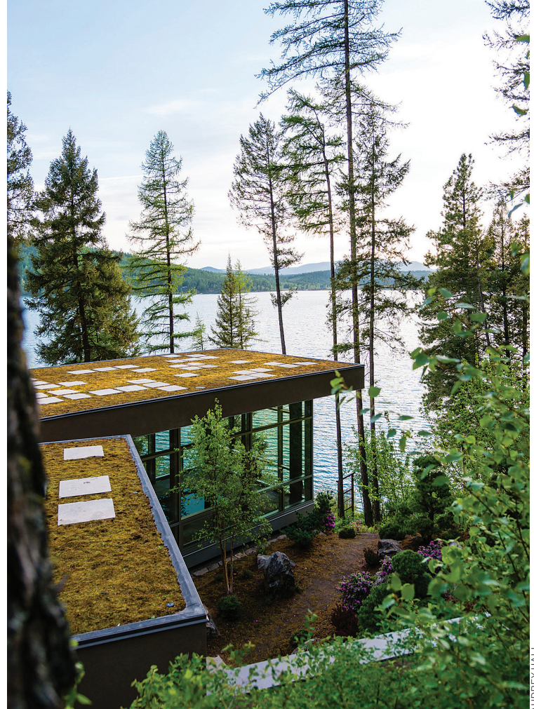
Perched on a steep slope above Whitefish Lake, this private pool-house design seeks to nest the small collection of buildings into the hillside, melding them into the natural contrasting grades.
